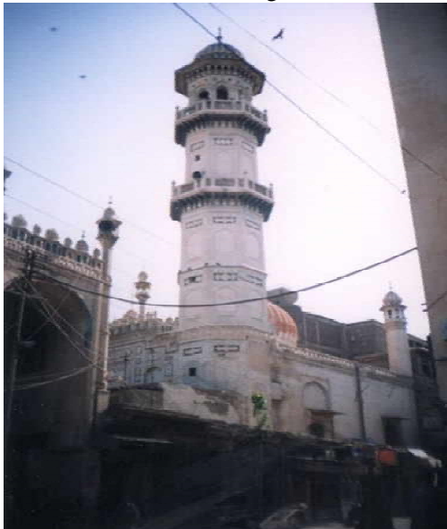
Figure 12: Minaret of Mosque Mahabat Khan constructed during the era of Mogul Emperor Aurang Zeb some 300 years ago. The minaret is about 60 ft high constructed in burnt brick masonry.
