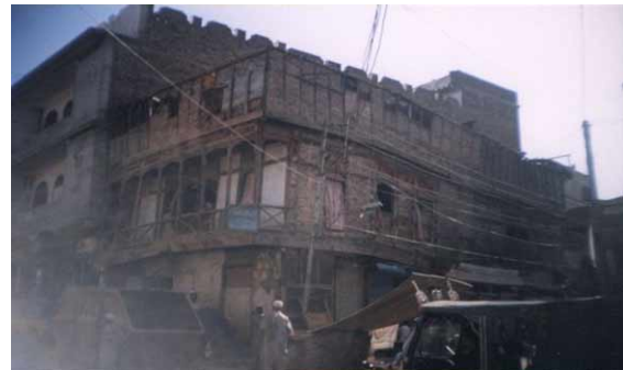
Figure 13: A 100 years old house constructed as wooden frame with un-burnt brick infill walls, situated in the center of the walled city
