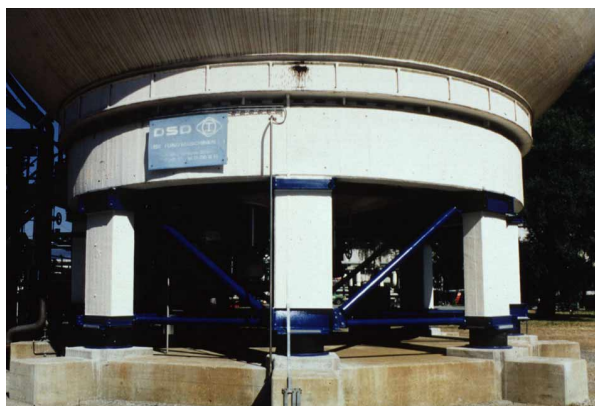
Figure 7: Insertion of high damping rubber bearings into RC columns for the seismic upgrading of liquid gas tanks: at column base (left) and at column top (right)
