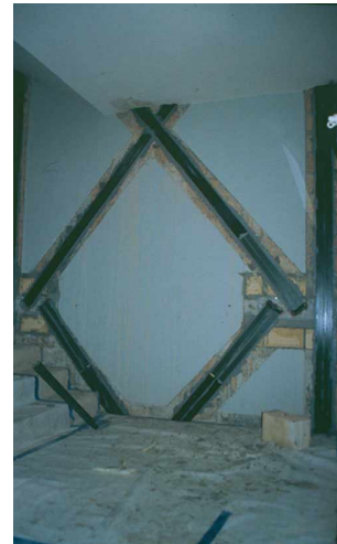
Figure 6: Truss-like CFP strips glued to URM walls and carefully anchored in the RC floor slabs (right) for the seismic upgrading of a 7-storey residential building (left)
