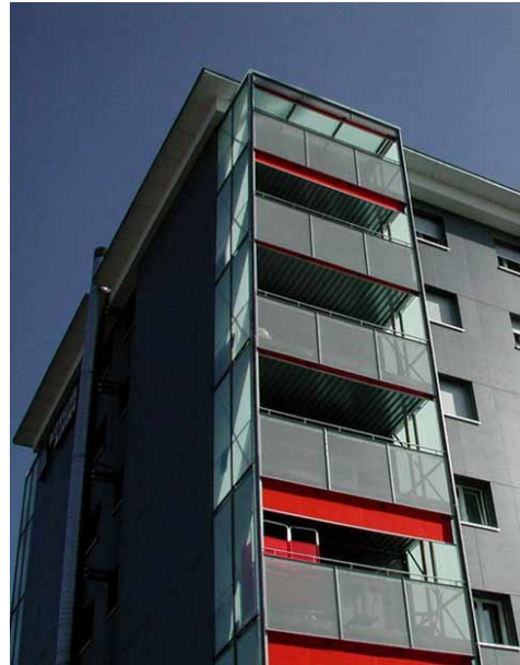
Figure 4: External RC structural walls for the seismic upgrading of three 8-storey residential buildings under construction (left) and after completion (right)
