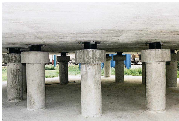
Figure 7: Insertion of high damping rubber bearings into RC columns for the seismic upgrading of liquid gas tanks: at column base (left) and at column top (right)
