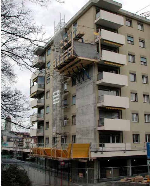
Figure 4: External RC structural walls for the seismic upgrading of three 8-storey residential buildings under construction (left) and after completion (right)
