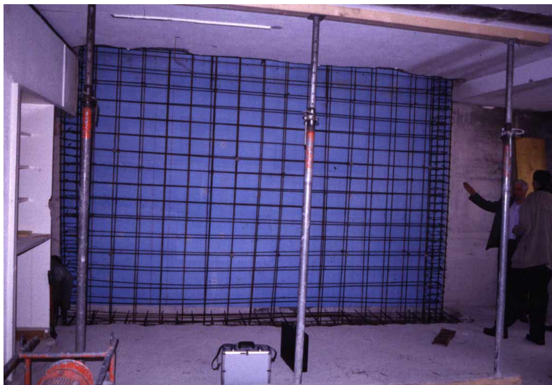
Figure 5: Internal RC structural walls for the seismic upgrading of a children's hospital
