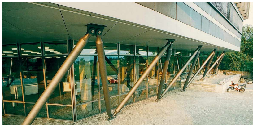
Figure 3: External inclined steel truss for upgrading an RC lecture theatre building for both, seismic actions and gravity loads
