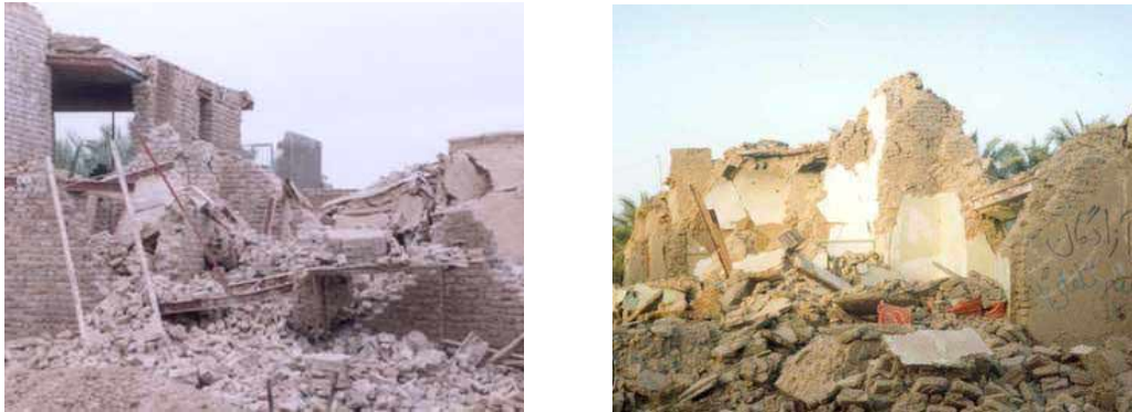
Figure 1. Iran earthquake, 26 December 2003. Collapse of vernacular houses in the city of Bam. ( www.ngdir.ir )
