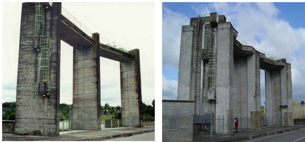
Fig. 4: Strengthening of crest spillway of the 56 m high Whakamura gravity dam in New Zealand (left: original design of 1956 with seismic coefficient of 0.1; right: strengthened structure with design acceleration of 1.9 g); Foster and Black (2003)
