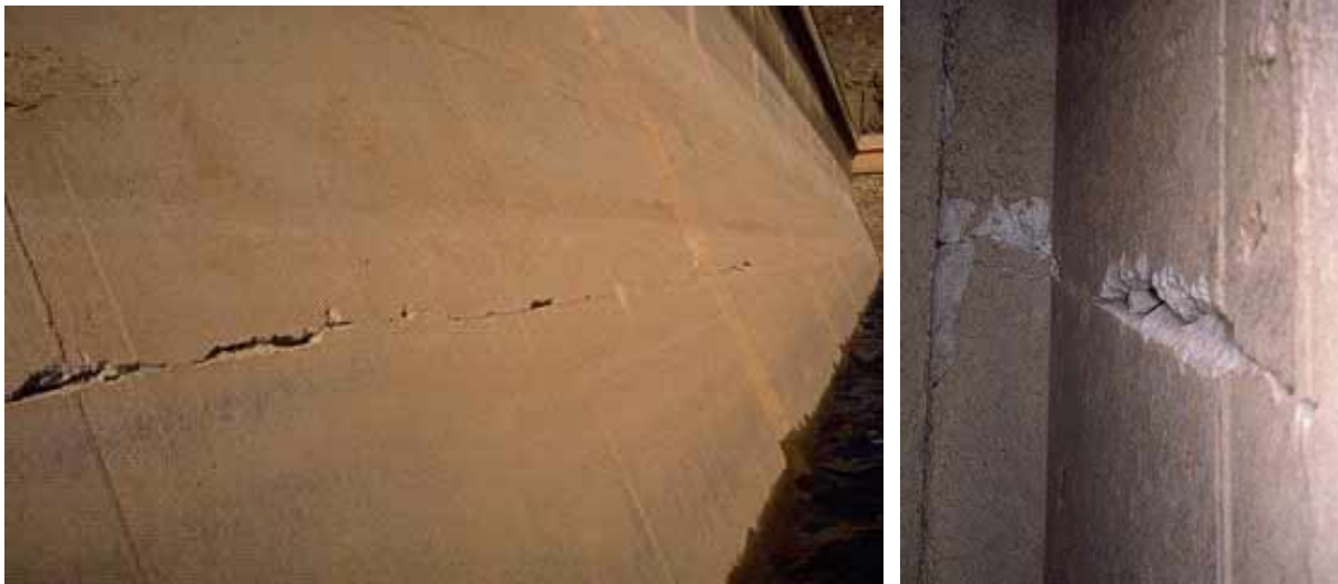
Fig. 1: Horizontal crack at lift joints in upper part of Sefid Rud buttress dam caused by 1990 Manjil earthquake in Iran (left: crack at upstream face across several buttresses; right: crack in web of buttress)
