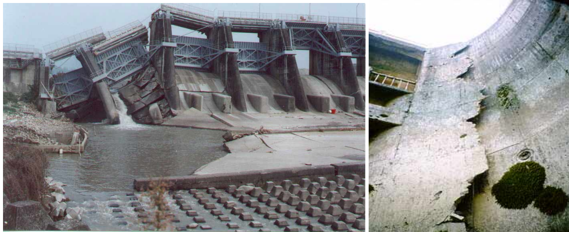
Fig. 2: Two bays of the Shih-Kang weir destroyed by fault movements during the 1999 Chi-Chi earthquake in Taiwan (left) and fault passing through intake structure (right)
