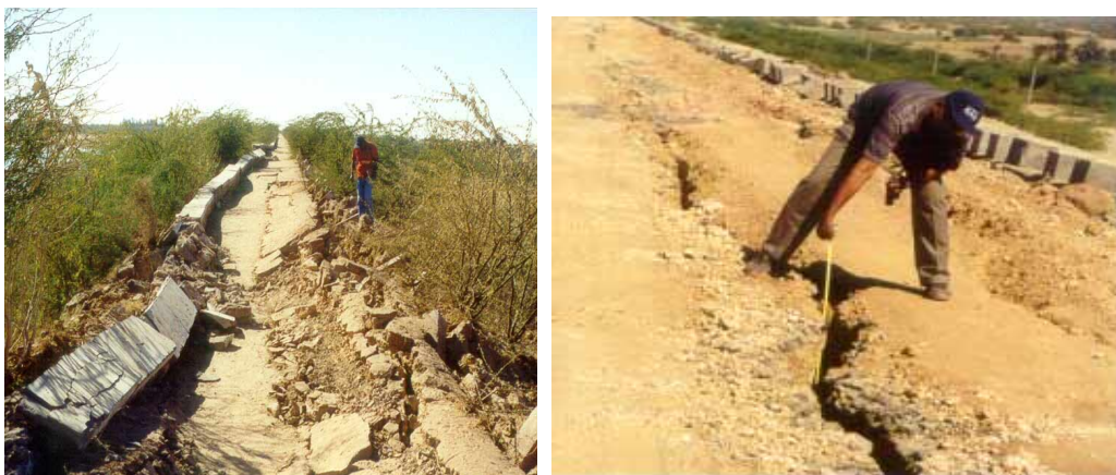
Fig. 3: Deformations in embankment dams caused by 001 Bhuj earthquake in India
