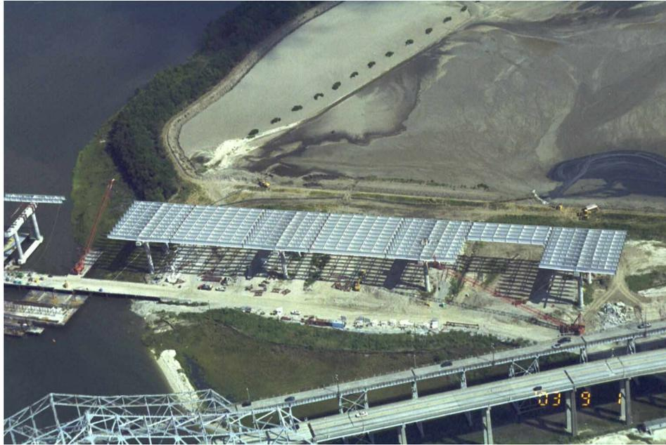
**Figure 13 – Erection of Steel Girders**
