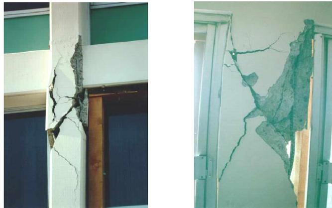
**Figure 14. Damage to Column C4 after Northridge Earthquake [17]**
