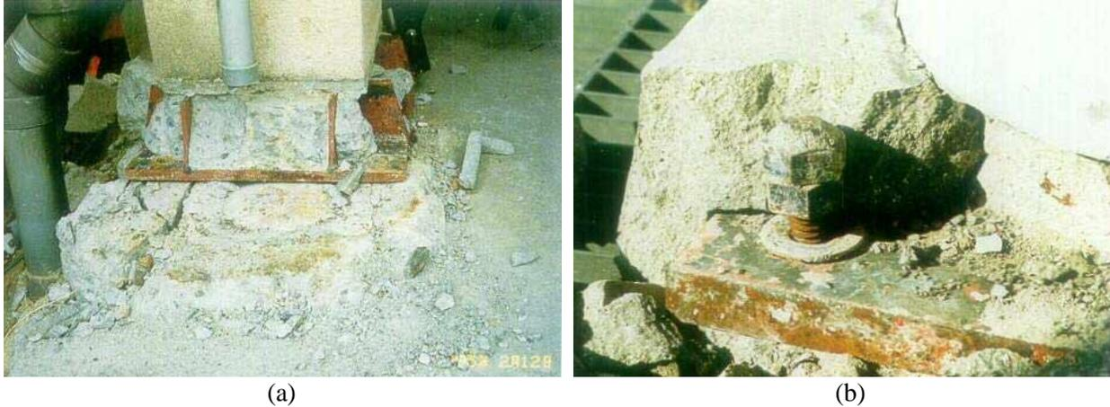
Figure 2: Column foundation damage: (a) Crushing of concrete pedestal of column-foundation joint due to pounding of base plate on the pedestal, and (b) Pull-out of anchor bolts and crushing of concrete pedestal at column-foundation joint during 1995 Kobe earthquake (AIJ, 1995). Pounding of base plate and pull-out of anchor bolts implies significant uplift of the base plate.
