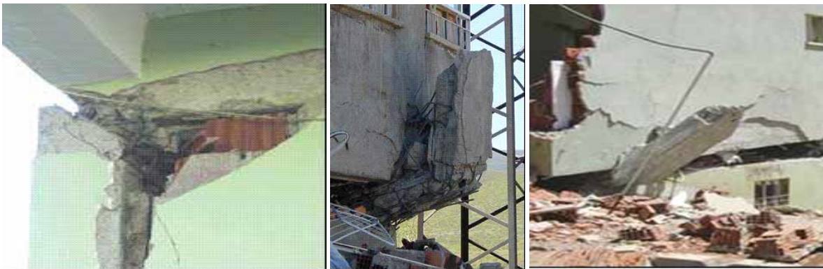
Figure 6 Column connection shear/dislocation in weak axes
