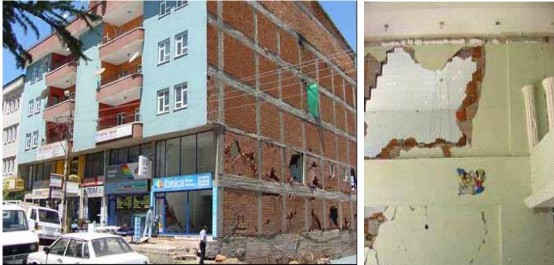
Figure 8 Infill wall damage
