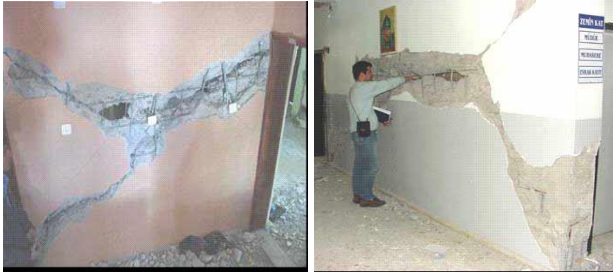
Figure 7 Heavy damage to shear walls
