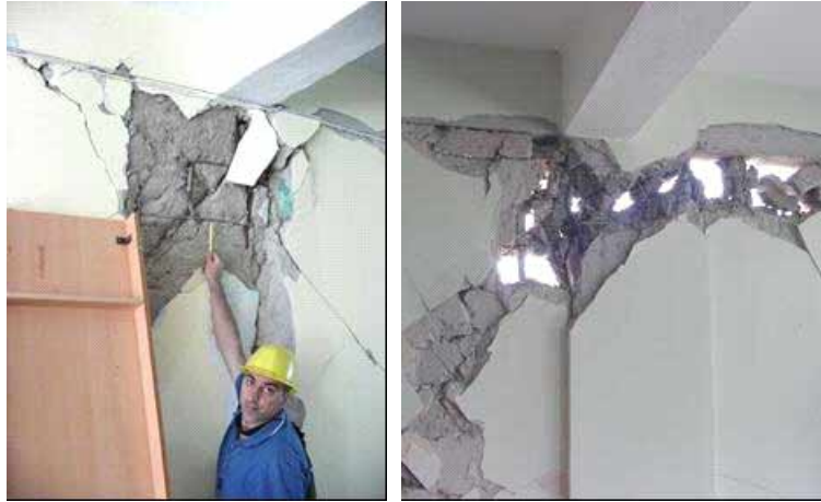
Figure 5 Column hinging and shear
