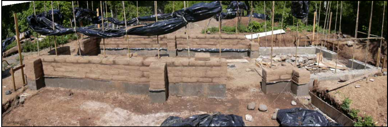
Figure 5. Adobe walls under construction, including plinth, pilasters, vertical reinforcement, plastic rain covers (Note: figure alignment offset due to photograph splicing).
