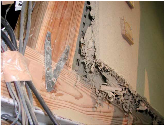
Photo 5 : [Plaster-wall test] Out-of-plane buckling of a plaster wall.
