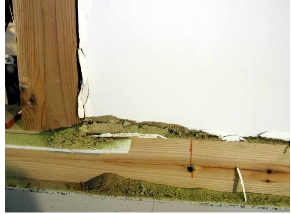
Photo 4 : [Plaster-wall test] Crumbling of a corner of a plaster wall.
