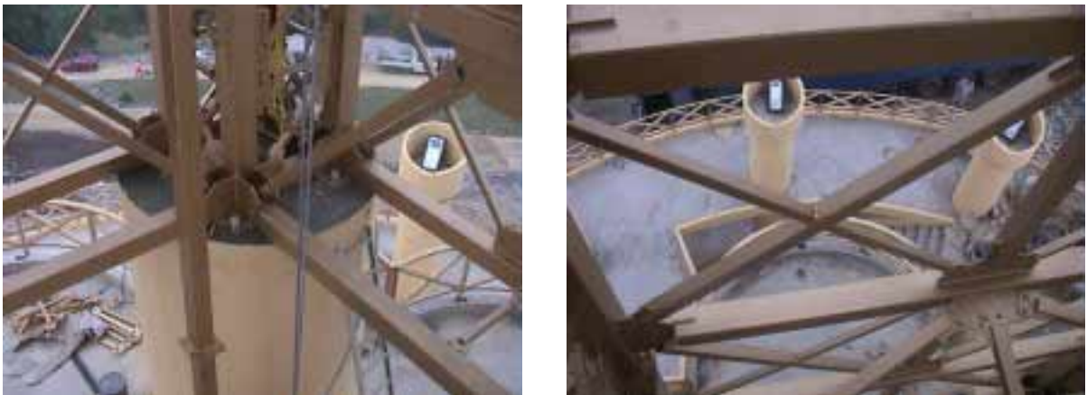
Fig. 13. Construction details: (a) resting of the corner of the vertical structure on the base and (b) joints of steel elements.
