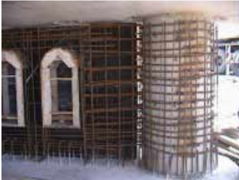
Fig. 9. Characteristic detail of construction of the RC structure of the pedestal
