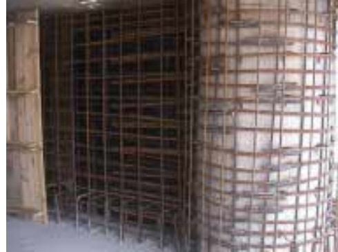
Fig. 9. Characteristic detail of construction of the RC structure of the pedestal
