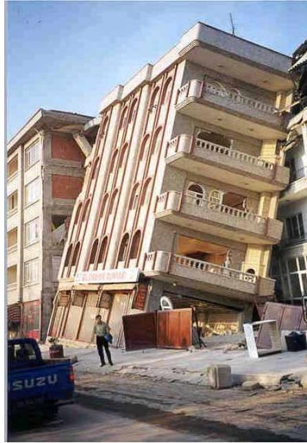
**Figure 1: Tilted building due to liquefaction in central Adapazari. Courtesy *Earthquake Engineering Field Investigation Team (EEFIT), UK***
