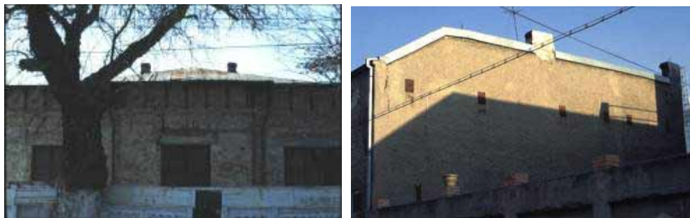
Figure 5: Wagon house; a) Typical damage; b) Retrofit with “ties” for “wagon” type house
