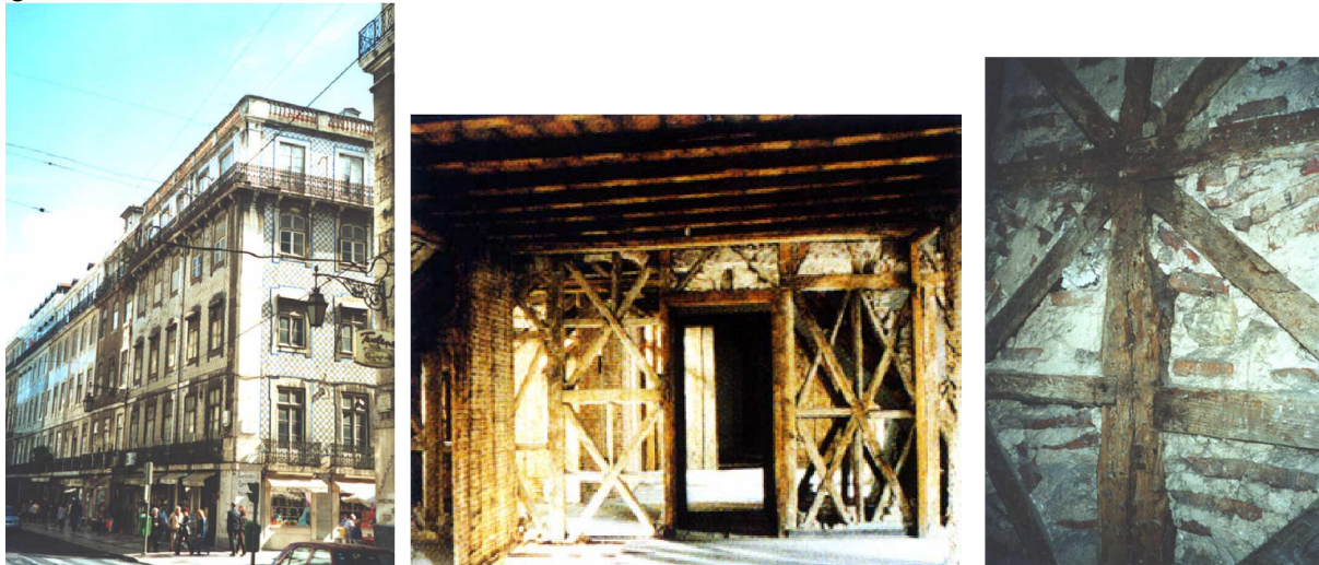
Figure 2: a) typical building block in the Baixa pombalina, Lisbon, Portugal; b) the cajola; c) cajola with infilled masonry
