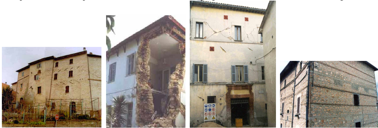
Figure 1: a) Typical array of Buildings in Nocera Umbra; b) corner failure in a building with stiff roof diaphragm (Greece) ; c) shear cracks on a wall with ties and stiffened vaulted floors (Nocera Umbra); d) introduction of concrete ring beam at each storey level (Nocera Umbra).
