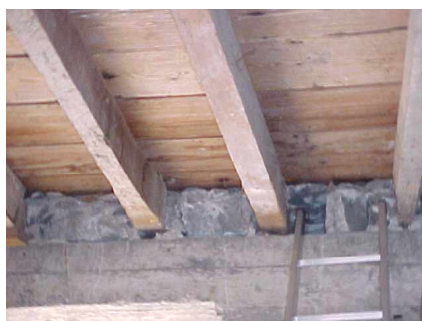
Fig. 8 – Detail of the floor supporting structure
