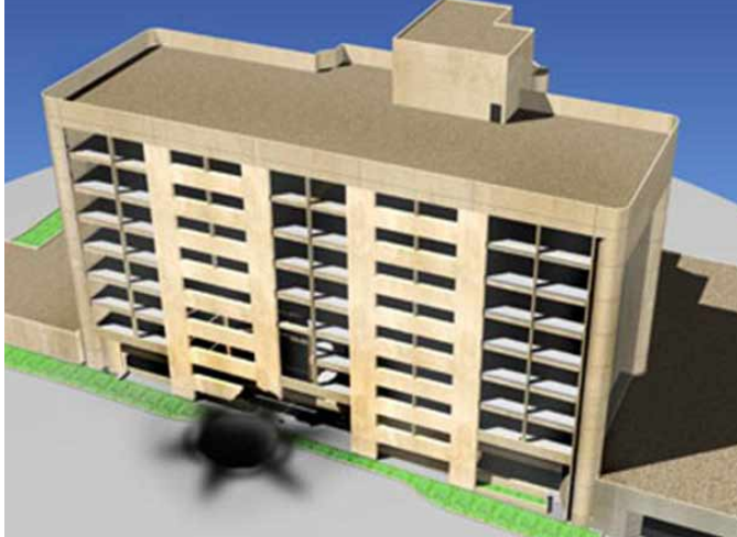
Figure 12 Estimated damage to pier-spandrel system in 1995 bombing scenario.
