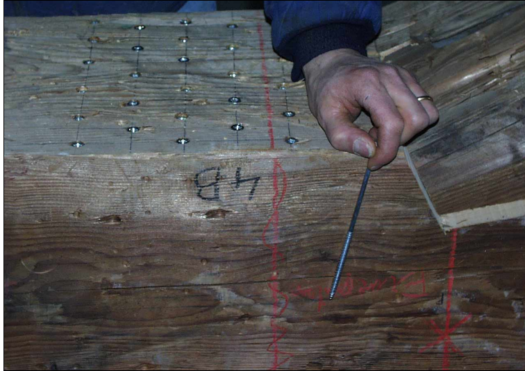
Figure 5. Simple and efficient reinforcement of the chord toe area, by means of metal screws
