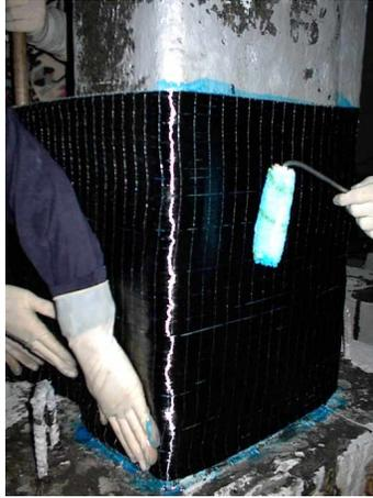
Figure 2. Application of CFRP sheets onto column surface
