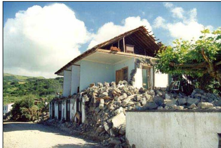
Figure 13 - Fall out the plane of exterior walls without complete collapse (1998 Azores earthquake)
