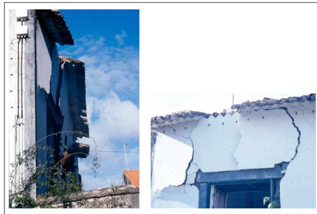
Figure 10 – Damages due to 1998 Azores Earthquake, similar to those obtained in the analysis
