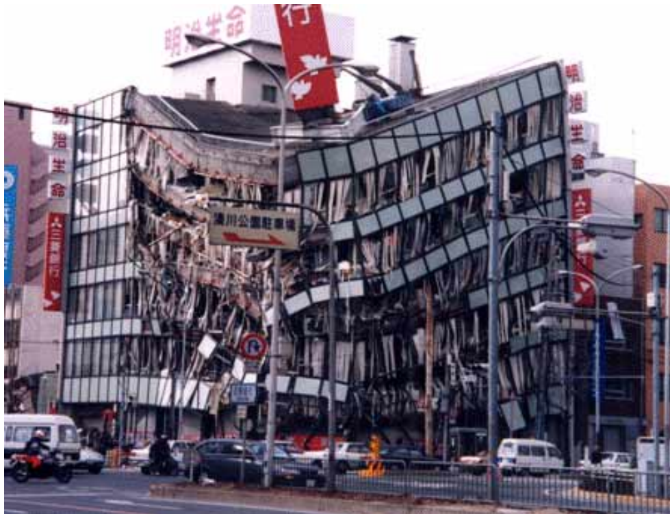
Figure 13: Collapsed steel building during January 17, 1995 Kobe Earthquake (by K. Meguro)
