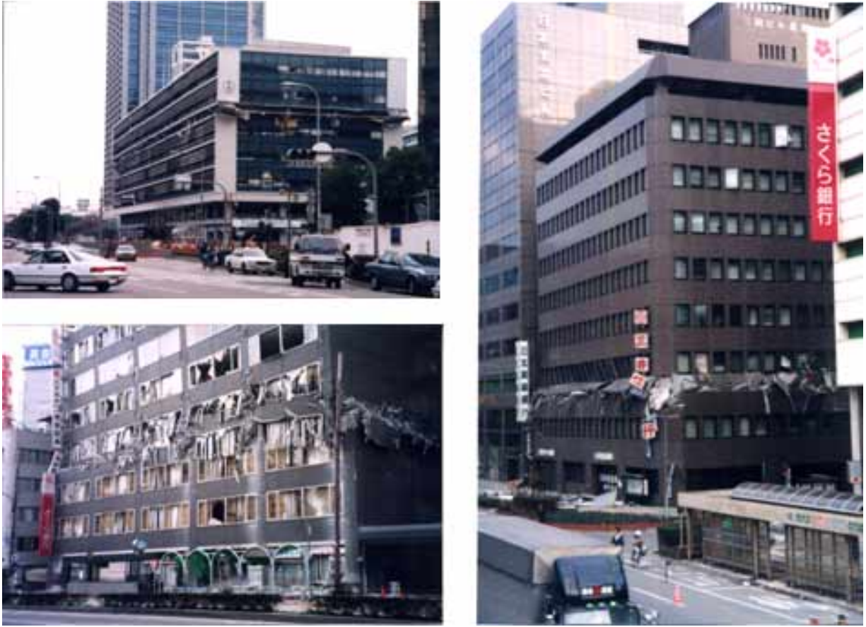
Figure 14: Collapsed commercial buildings during January 17, 1995 Kobe Earthquake
