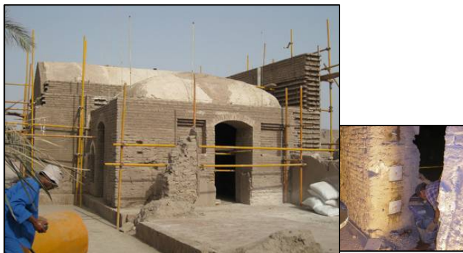
Figure 9 Strengthening of the Sistani House, by Dresden University of Technology-Germany
