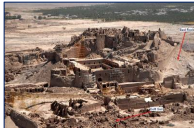
Figure 3 The bed rock in District of Governor caused different dynamic response in comparison with other parts
