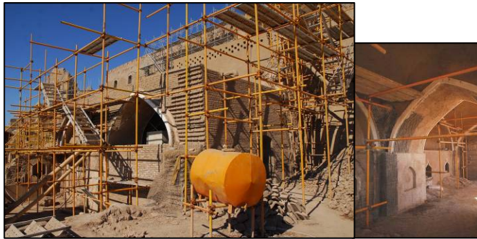
Figure 8 Strengthening of the Stable, by SES Consulting Engineers, Iran
