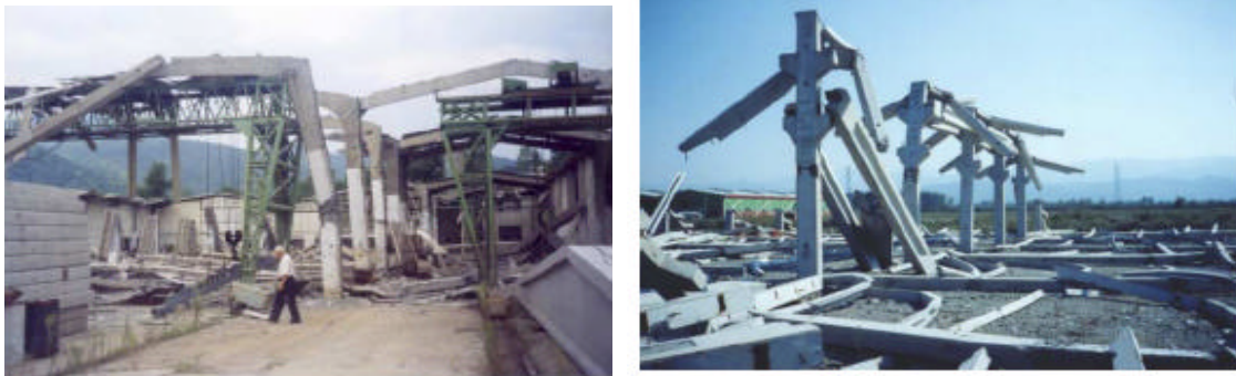
Figure 3 Overall collapse of the prefabricated systems
