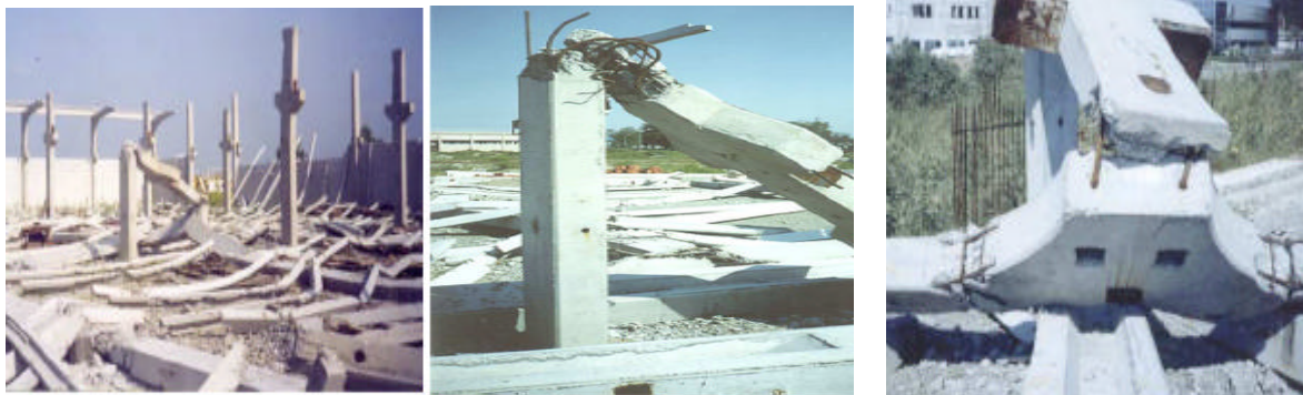
Figure 4 Seismic damage of the system
