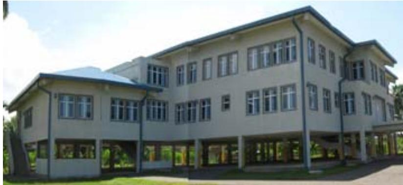
Figure 1 A tsunami resistant building with elevated lower level in Sri Lanka
