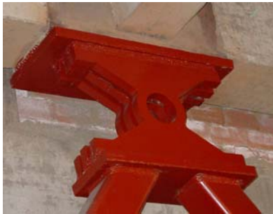
Fig 11 (a) Installation of single round-hole damper Fig 11 (b) Installation of double X-shaped damper
