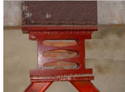
Fig 11 (a) Installation of single round-hole damper Fig 11 (b) Installation of double X-shaped damper
