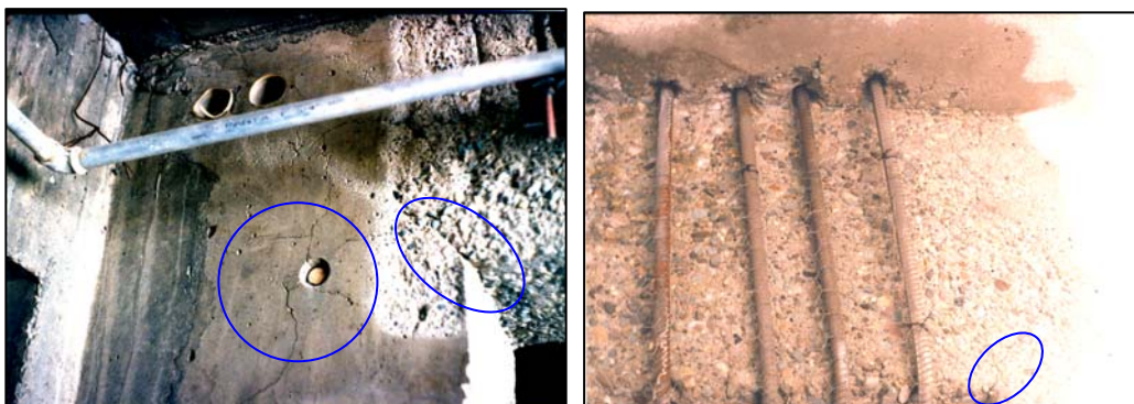
Figure 7 – Structural cracking of a coupling beam in middle stories after sand blast
