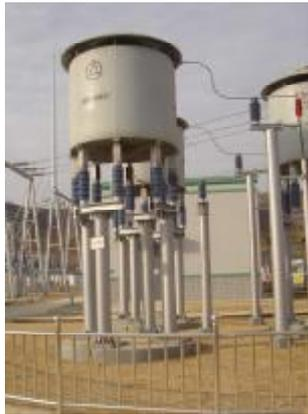
Figure 4 Picture of High-voltage reactor
