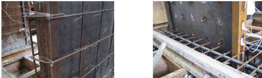
(a) reinforcement grid and steel channel (b) shear studs welded on the steel plate
