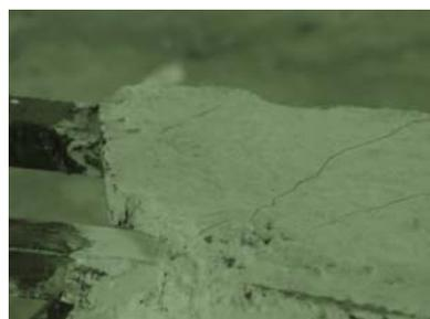
Figure 4 Cracks between the steel truss and Core1
