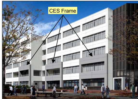
Figure 1 Concept of the RC frame externally retrofitted by CES frame
