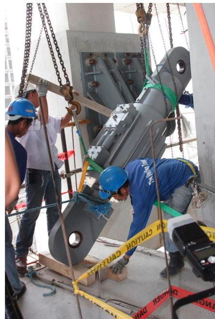
Figure 5 Installation of Dampers
