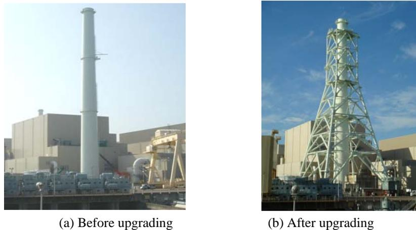
Figure 1 Photo of the stack (unit-4)
