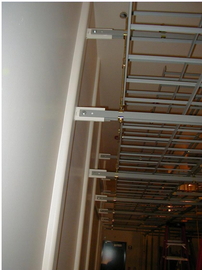
Figure 5 Typical HSS Bracing Members Attached to Proprietary Channels
