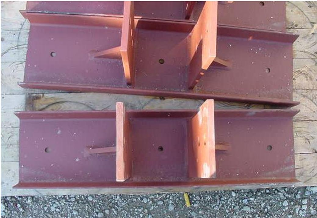
Figure 6 Custom brackets used to attach the top of the HSS bracing elements to the roof
