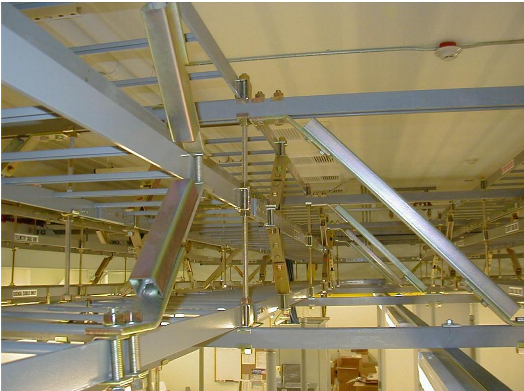
Figure 3 Typical configuration of layers of cable trays supported on proprietary steel channels
