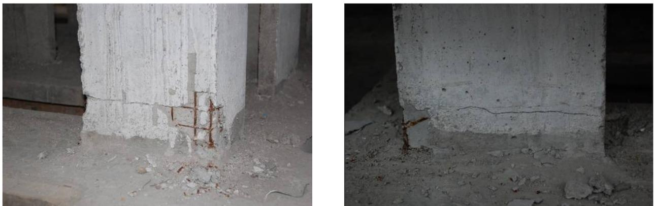
Figure 7: Concrete crack on the bottom of the shear wall
