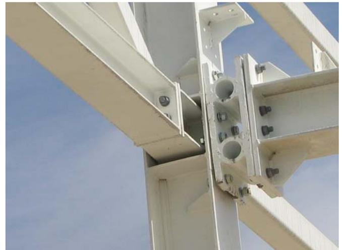
Figure 23- A real application of KHONSAR™ connection, during the course of installation of the structure.
