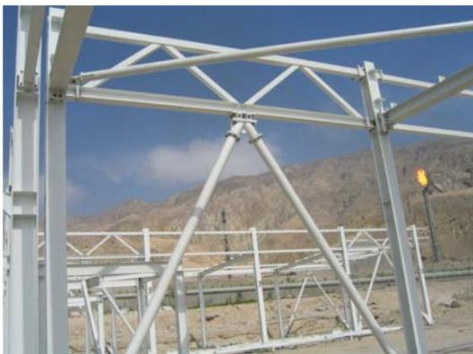
Figure 23- Application of KHONSAR™ as a brace-to-frame connection.
