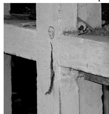
Figure 5 Concrete spall near joints
