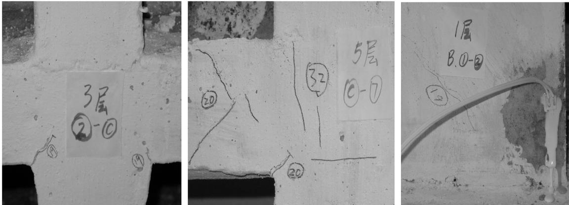
(a) Oblique crack in beam-column joint
