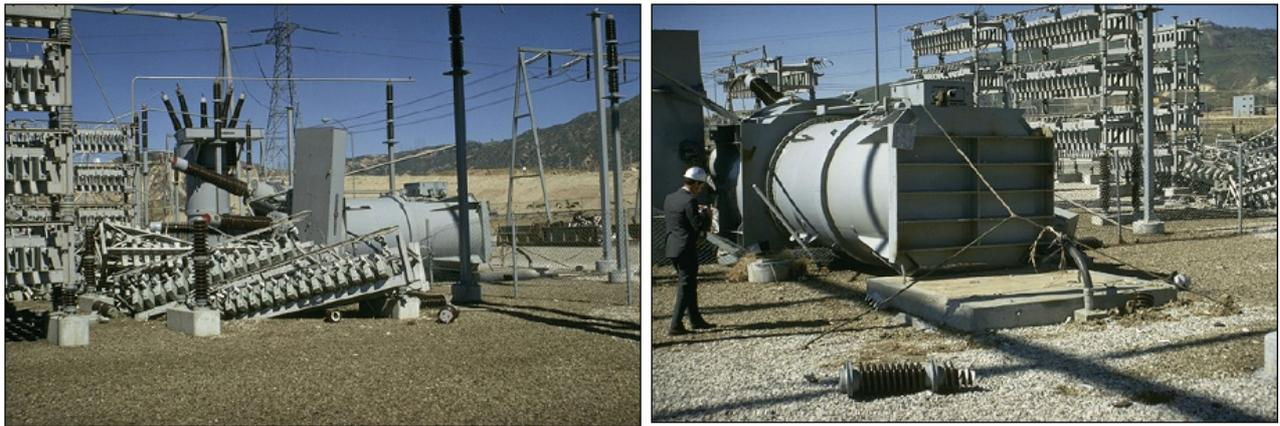
Figure 2 An electrical transformer at the Sylmar Converter Station, California that overturned during the 1971 San Fernando earthquake (by Makris, 1998).
