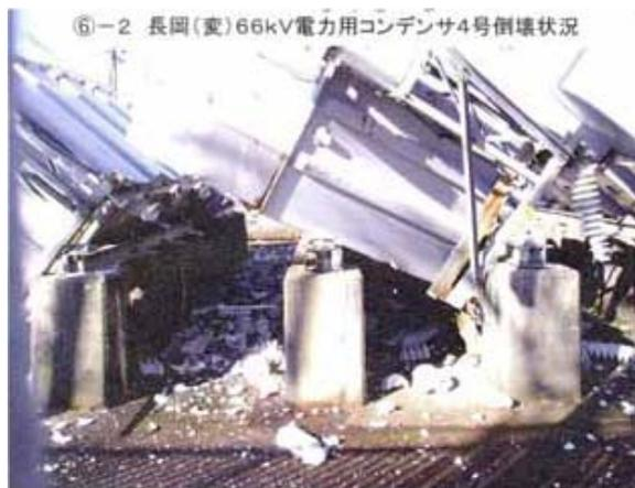
Figure 3 Failure of condenser in Nagaoka sub. (JSCE, 2004)
