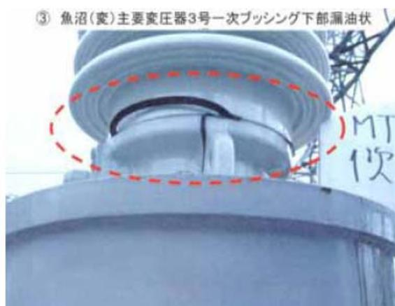
Figure 4 Extrusion of gasket and oil leakage in bushing of 154 kV transformer in Uonuma Sub. (JSCE, 2004)
