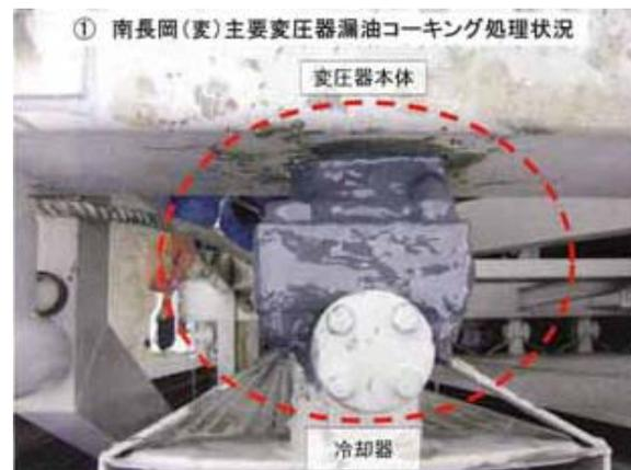
Figure 2 Oil leakage from joint between transformer and condenser in Minami Nagaoka Sub. (JSCE, 2004)
