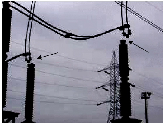
Figure 4: A flexible clamp
