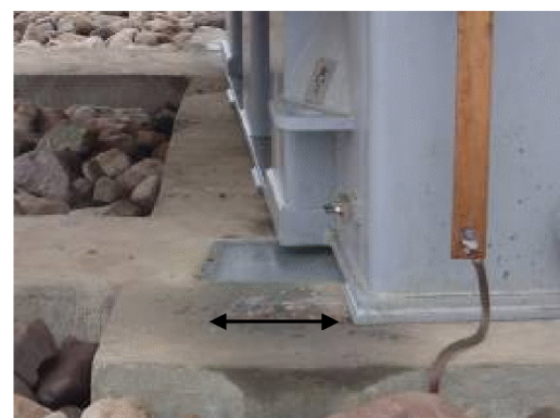
Figure 7: Sliding of non-anchored equipments
