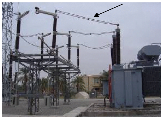
Figure 6: Pulled conductor
