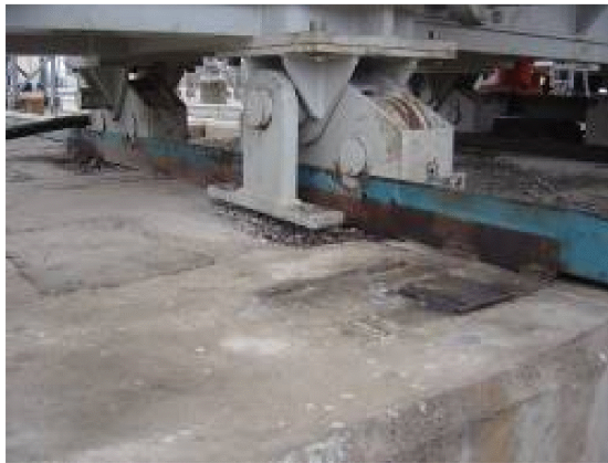
Figure 10: Transformer base after retrofit
