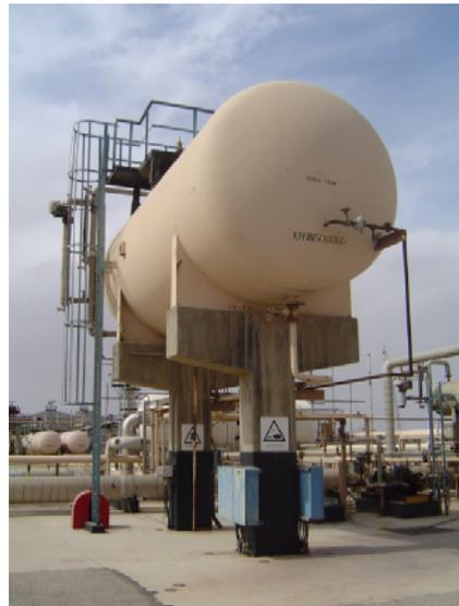
(b) - A typical of horizontal pressure vessel
