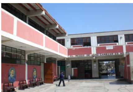
Fig. 8- The school building on the left, designed with the 1977 Seismic Code suffered short-column failure. The one on the right, designed with the 1997 SC was undamaged.
