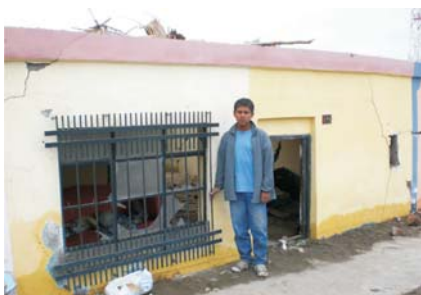
Fig. 2- One-story brick masonry house settled some 0.70 m
