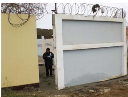
Fig. 6- These two portions of wall were aligned, separated by only 2 cm. An employee of the town hall is seen through "the door opened" by lateral spread.
