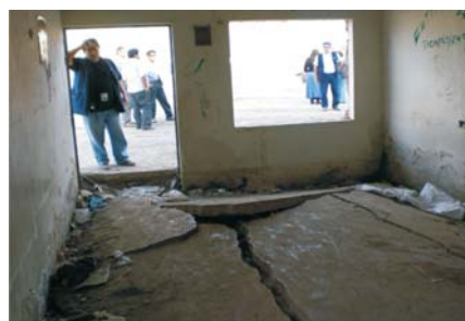
Fig. 3- Notice that the walls have sunk some 0.40 m, and the floor 0.20 m
