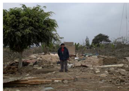
Fig. 9- Over 40,000 adobe houses collapsed mostly in rural areas irrigated by inundation. Entire blocks of houses collapsed in Sunampe, Chíncha and in Hualcara, Cañete.
