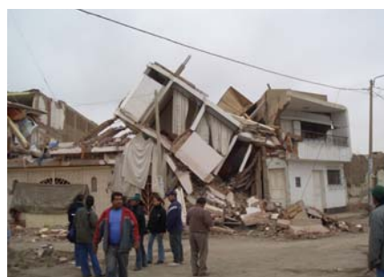
Fig. 7- Collapse of a reinforced concrete building in downtown Pisco.
