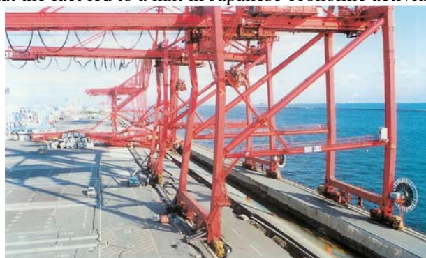
Fig.1 Destroyed container crane on quay wall at Kobe Port (1995 Hyogoken-nambu Earthquake)
