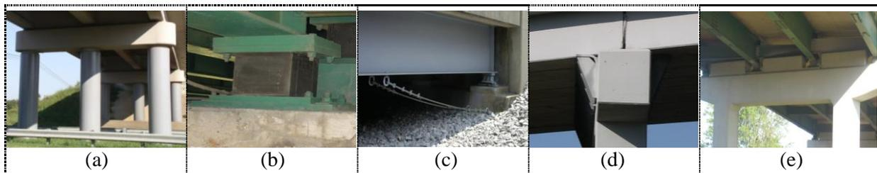
Figure 2 Bridge retrofits considered: (a) steel jackets, (b) elastomeric isolation bearings, (c) restrainer cables, (d) seat extenders and (e) shear keys
