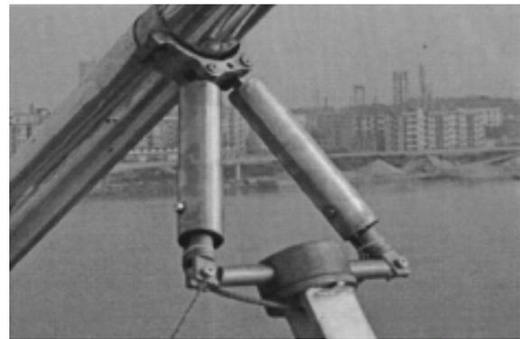
Figure 7. MR damper installed on the Dongting Lake Bridge in China.
