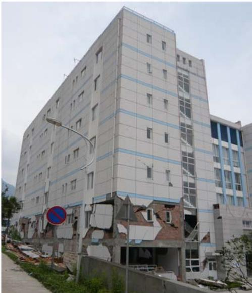
Fig. 3 Shear crack of the bottom two stories of an office building in Dongfang Steam Turbine Works, Hanwang town, May 15, 2008
