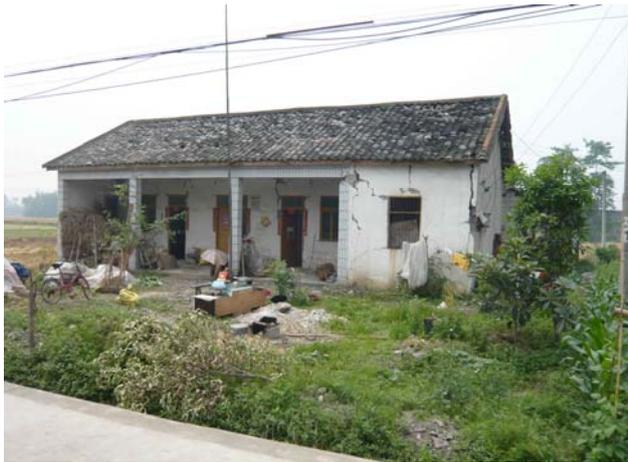
Fig. 13 A moderate destroyed rural house with severe cracked walls, Mianyuan town, May 16, 2008
