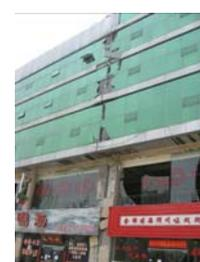
Fig.27 Damage and falling of glass curtain walls resulted from collision of the seismic joint
