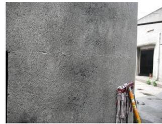
Fig.22 Cracks at root of the water tower structure
