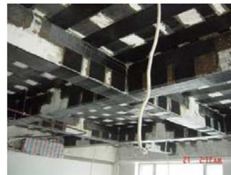
Fig.31 Reinforcement of beam and slab by pasting carbon fiber sheet
