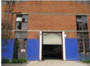
Fig. 8 Masonry cracks at the door opening have been reinforced with steel frame
