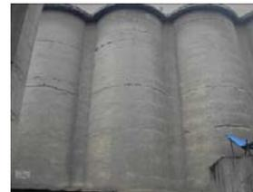
Fig.24 Circular cracks and displacements at mid height of multiple cement bunkers
