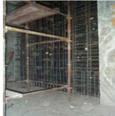
Fig.41 the added RC shear wall
