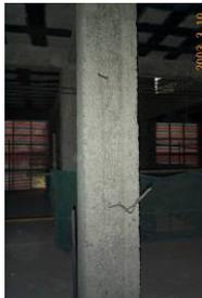
Fig.37 Roughening of the surface of the original concrete column
