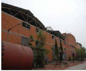
Fig. 6 Gable masonry of plant buildings with ring-beams partially collapsed
