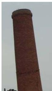
Fig.19 Circular cracks in the upper middle part of the chimney
