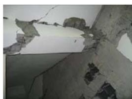
Fig.13 Stair girder, pillar damaged
