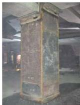
Fig.33 Reinforcement of column by wrapping steel plate
