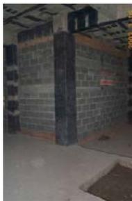
Fig.30 Reinforcement by wrapping carbon fiber sheet around the column
