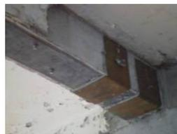
Fig.34 Reinforcement by pasting steel plates on the bottom and sides of the beam
