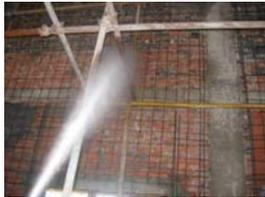
Fig.40 reinforcement of the masonry of a hotel building in Beijing with shotcrete
