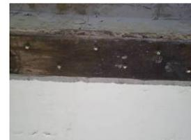
Fig.35 Steel plate is fixed by using chemical anchoring bolts
