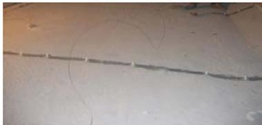
Fig.28 Pressurized grouting into cracks
