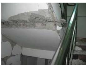
Fig.12 Stair carriage broken
