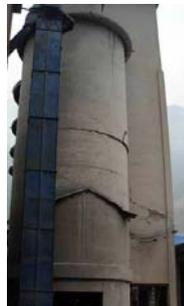
Fig.23 Circular cracks and displacements at mid height of individual cement bunker
