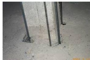
Fig.38 Longitudinal rebars of the column threading through the floor slab
