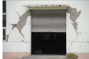
Fig. 9 Masonry at door opening with rain shed cracked
