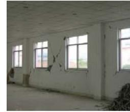
Fig.16 Masonries of partition walls at windows openings have X-shaped shearing cracks
