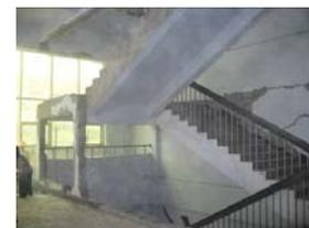
Fig.14 Stair partition wall totally collapsed
