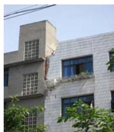
Fig.26 Partial collapse resulted from collision of buildings on both sides of the seismic joint
