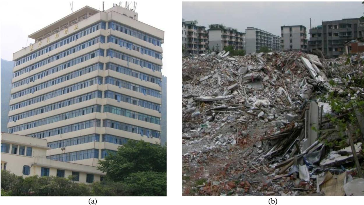
Figure 4: Building damage in the area of the Oriental Turbine factory: (a) an office RC shear wall building with slight to moderate damage, (b) residential CM buildings collapsed (front) and severely damage (rear)
