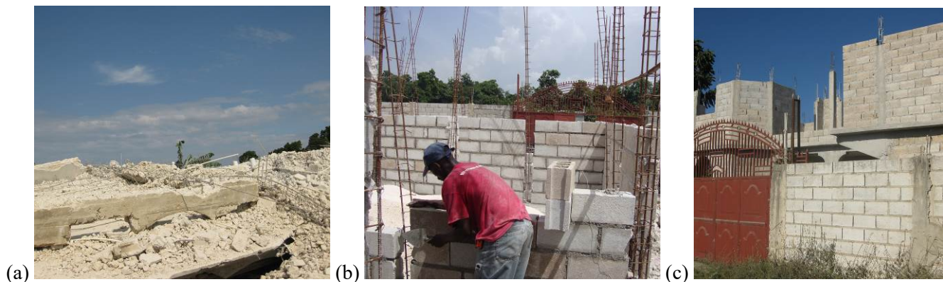
Fig. 2. Time lapse of heavily partitioned home with CMU load-bearing walls that experienced (a) pancake collapse in Léogâne, [documented in March 2010], (b) undergoing reconstruction in August 2010 following re-education of the head mason [documented in August 2010], and (c) continuing to a second floor with many of the same principles that created the original vulnerabilities [documented December 2011].
