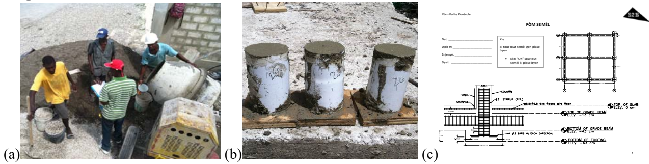
Fig. 8. (a) A quality control engineer using a visual checklist for concrete production, (b) concrete samples cast with design concrete mixes to prove increased strength to crews, (c) sample visual quality control form
