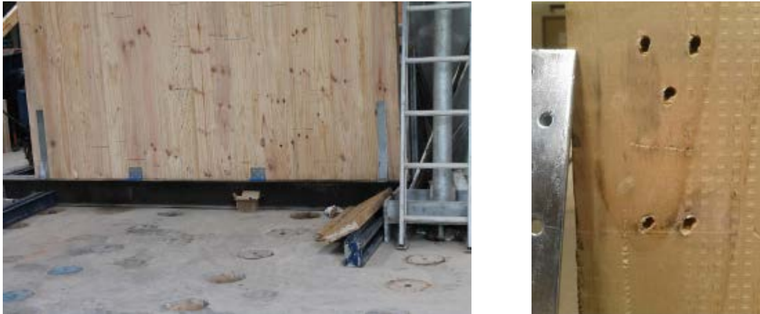
Figure 5: Tested wall supports layout (left). Timber crushing on hold down fasteners holes (right)
