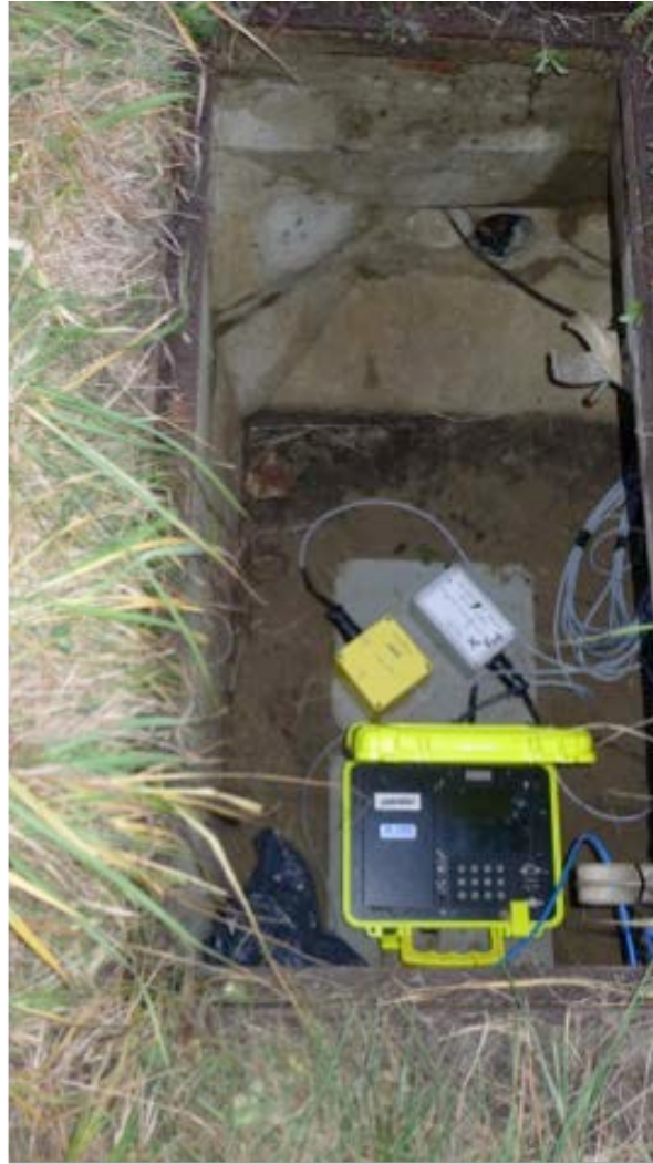
Fig. 2 – Instruments deployed in the vault
