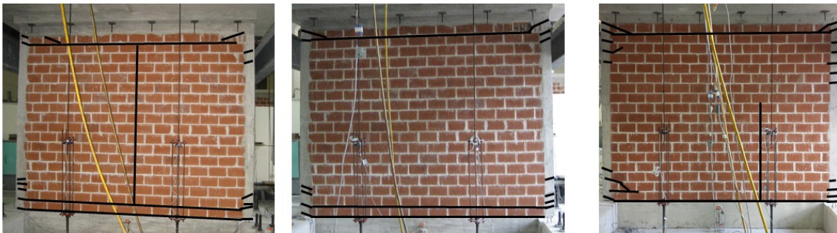
Fig. 3 – Final cracking patterns of walls
